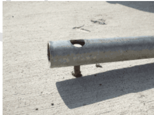
Figure 9: Poorly Anchored Bike Rack
