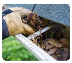
Eavestroughs should be checked and cleaned twice annually, in the spring and fall. Clear out any debris to ensure that rain and snow melt can flow freely. During a rainfall event, look to see if your eavestroughs are sagging or leaking anywhere. A sagging eavestrough will likely need to be replaced. Leaks can often be filled with caulking
