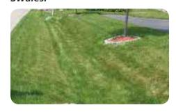
A swale is a shallow vegetated channel, often located along property lines, that collects and drains stormwater. Swales should be maintained by regular mowing and clearing any debris that could block the passage of water.
