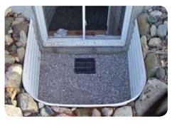
A properly installed window well on any basement window will help to ensure that water infiltrates into the weeping tile while preventing seepage into your home. Window wells are inexpensive and easy to install.
