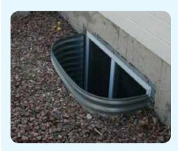
Measure your window to ensure that you buy the correct size window well. The window well should fit firmly against the foundation wall with the edges fitting comfortably around the window.
