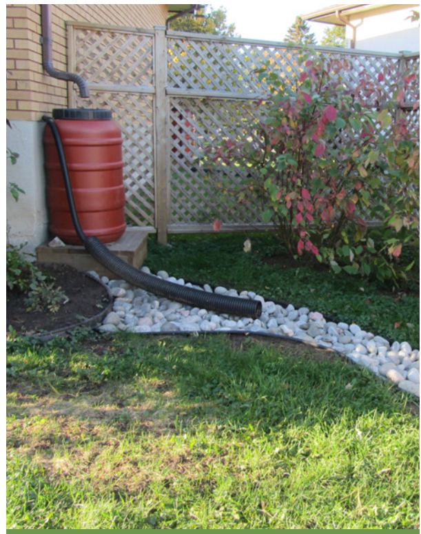
Overflow water from a rain barrel is directed into a swale lined with river rock.
